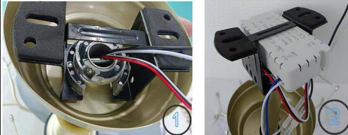
Step 8:snap the light body into the pegboard and put the driver into the pegboard slot.
